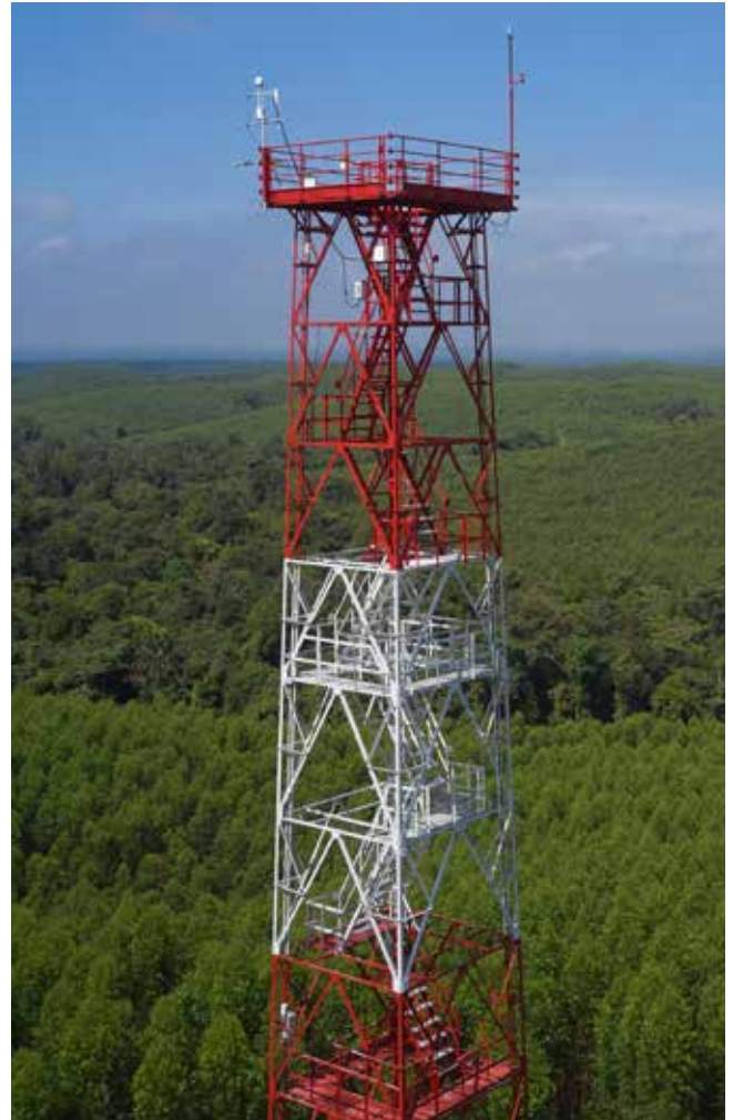
One of the four flux towers, which are used for the measurement of GHGs, on APRIL's, concession areas
